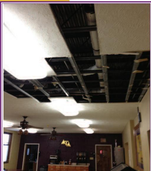
The dining room ceiling is exposed to make room for new plumbing, electrical, and fire-safety systems.
