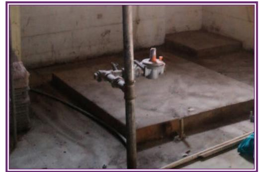
*A view of the concrete pad in the laundry room where the old boiler used to sit. In removing the boiler, an underground fuel tank that served as a secondary fuel source was discovered. The tank needs to be drained and removed, adding additional expense to the project.*
