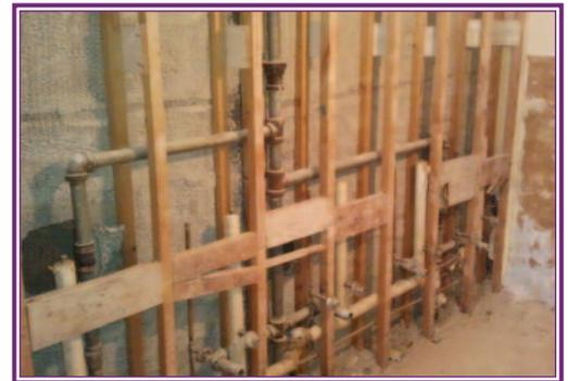
*New sink fixtures, flooring, wall finishes, toilet partitions, and showers will be installed in the second-floor bathroom. After uncovering all of the plumbing, we found some pipes that have been leaking for years which will now be repaired.*
