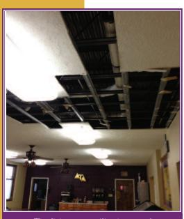
The dining room ceiling is exposed to make room for new plumbing, electrical, and fire-safety systems.
