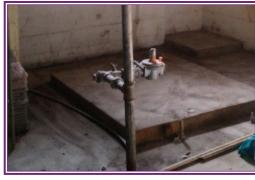
A view of the concrete pad in the laundry room where the old boiler used to sit. In removing the boiler, an underground fuel tank that served as a secondary fuel source was discovered. The tank needs to be drained and removed, adding additional expense to the project.
