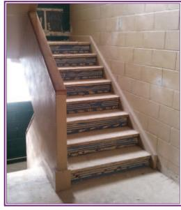
The stairwells on the west side of the house will receive new rubber stair treads and risers, new handrails, and the walls and ceilings will be repainted.
